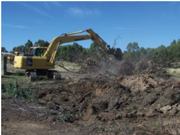
Figure 9. An excavator removing large woody weeds from Happy Valley Road site (P127499), December 2009 (Calum Walker).
